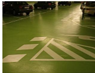
*This system is up to the mechanical and chemical stresses caused by car traffic. It is resistant towards mineral oils, fuel and skid-marks. Furthermore it satisfies the demands regarding anti-slip properties.*
